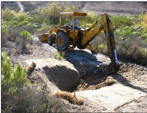
Erosion control through construction of sediment traps
