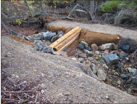
Erosion control using log dam, rock and fabric
